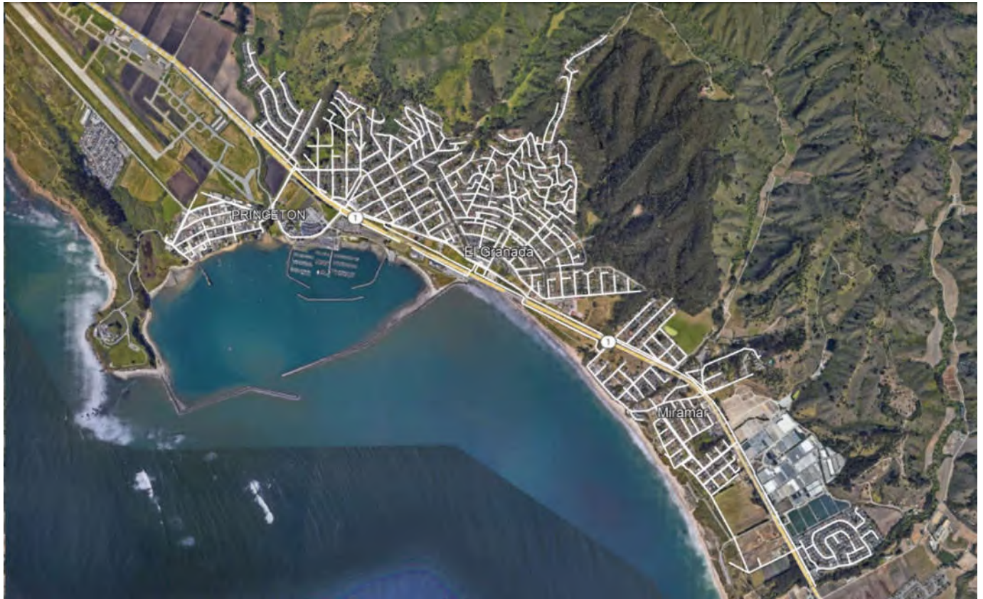
Figure 4-1 GCSD Sewer Pipelines
