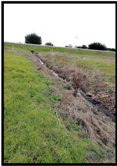
Figure 9.0: View facing southeast toward Drainage Ditch 1
