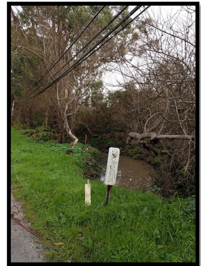
Figure 9.2: View facing southeast of Burnham creek.
