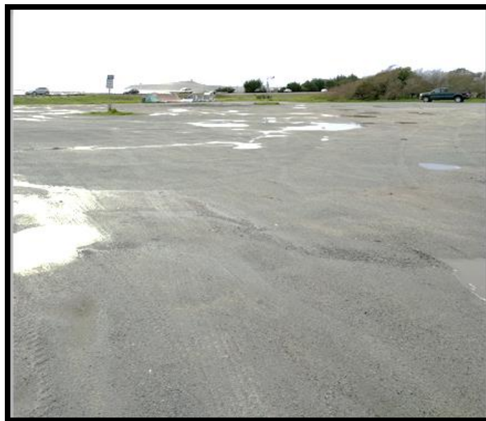
Figure 7.1: View facing southwest of the compacted area.
