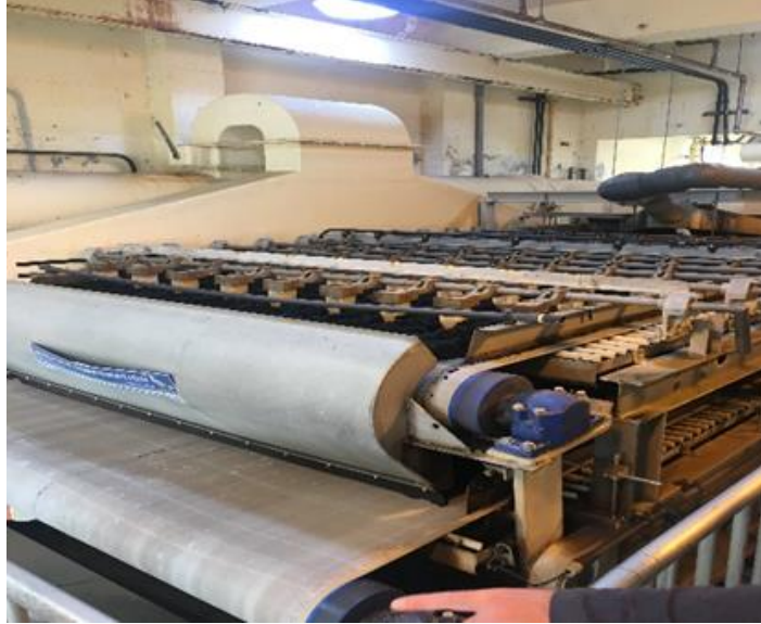
Figure B-11 Belt Filter Press
